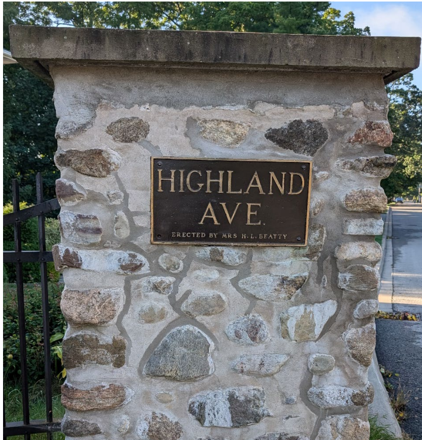
Figure 3- Highland Avenue Column
