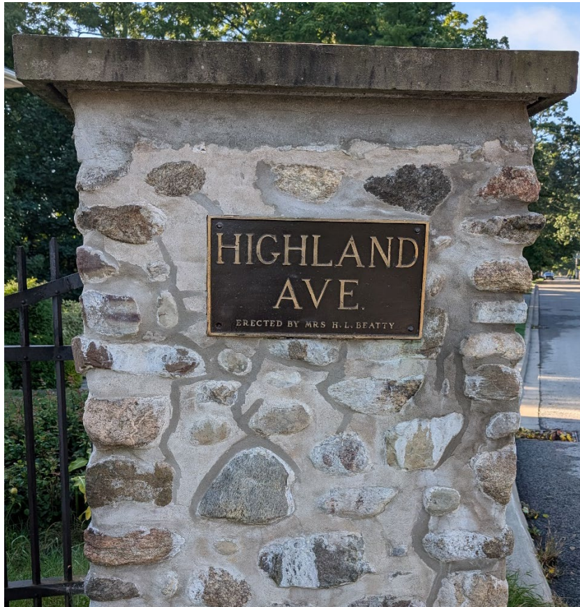
Figure 3- Highland Avenue Column
