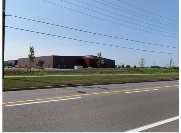
VIEW WEST AT THE NORTHERN PORTION OF THE SITE
