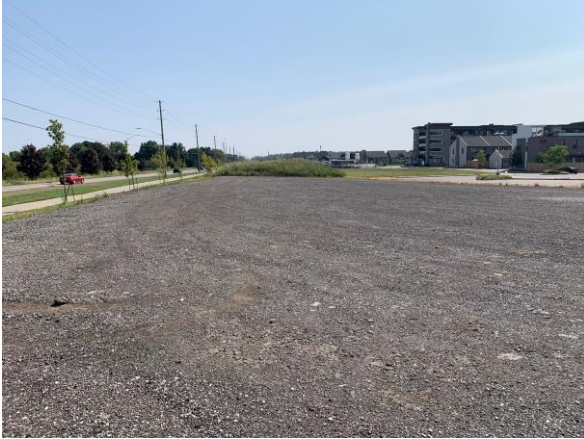
VIEW LOOKING SOUTH FROM THE NORTHEAST CORNER
