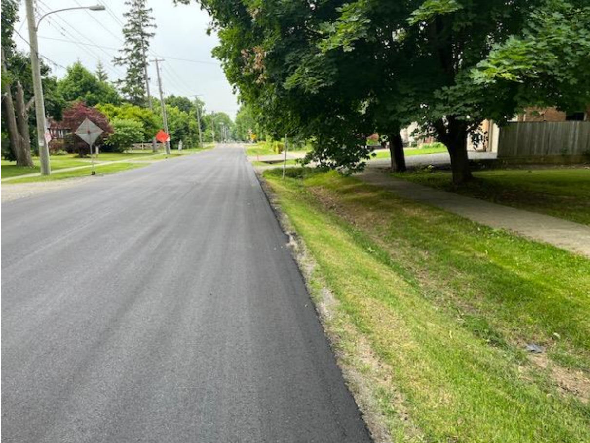
Church Street, North of the tracks, southbound approaching crossing.
