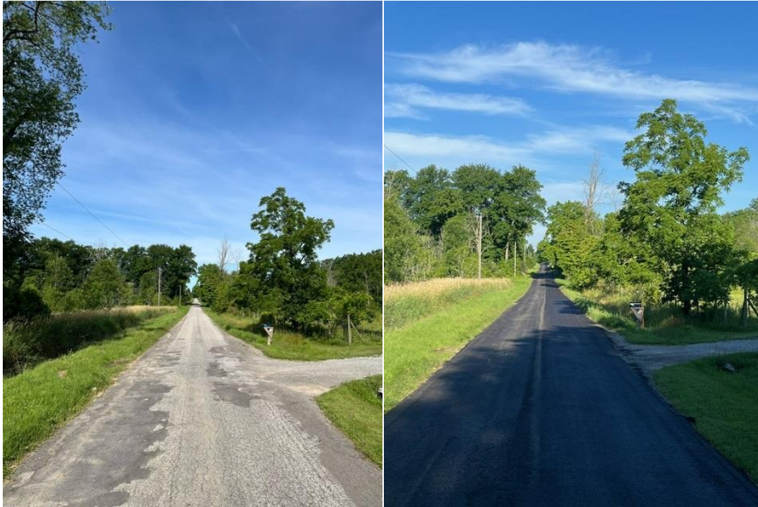
Kilman Road between Maple Street and Victoria Ave, before and after
