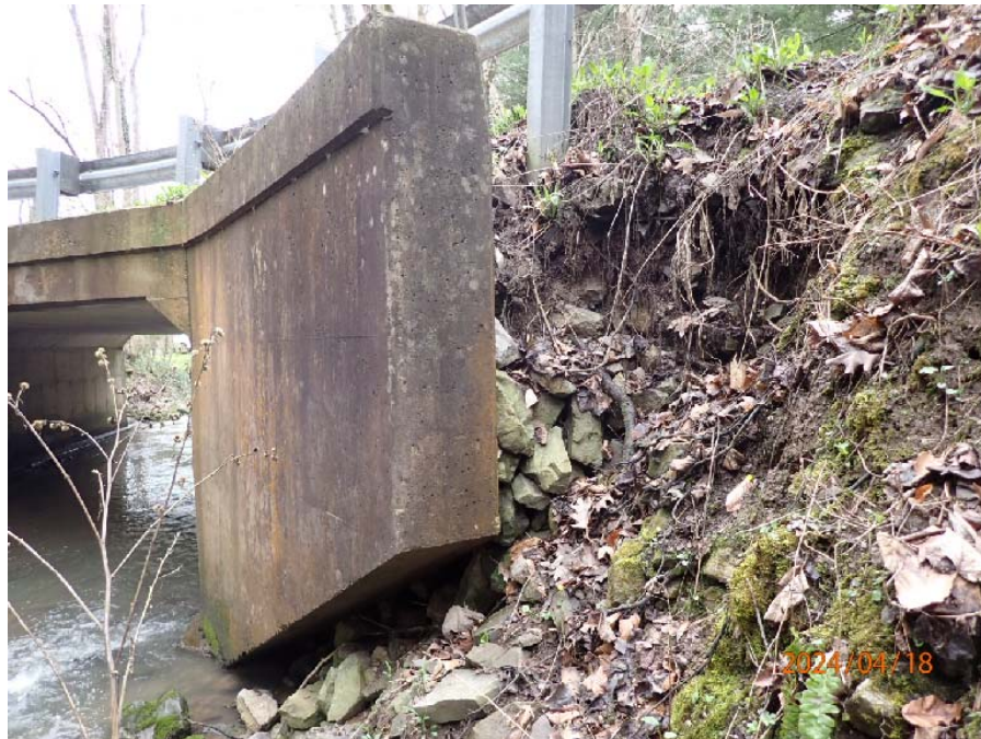
Photograph No. 4: 0571: Erosion at northwest wingwall.
