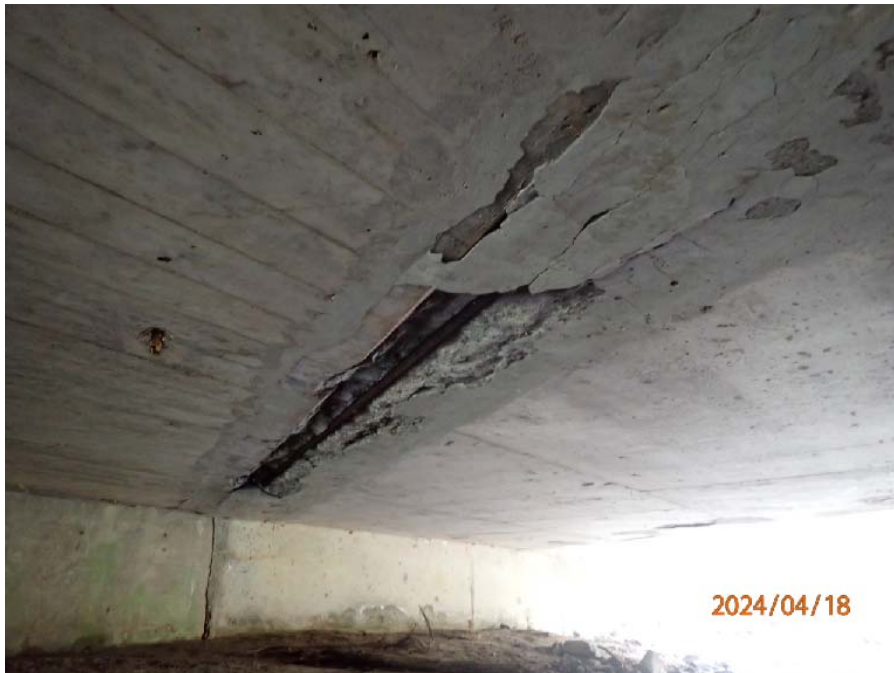
Photograph No. 4: 0326: Area of spalling and delamination at centre span, looking south.
