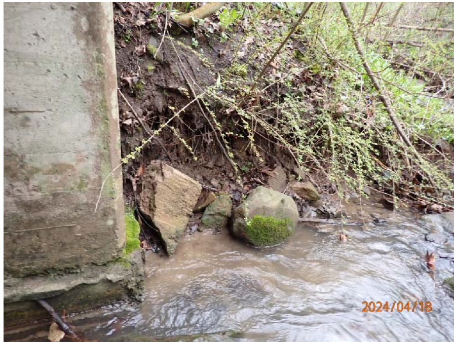
Photograph No. 4: 0405: Erosion at northwest corner.
