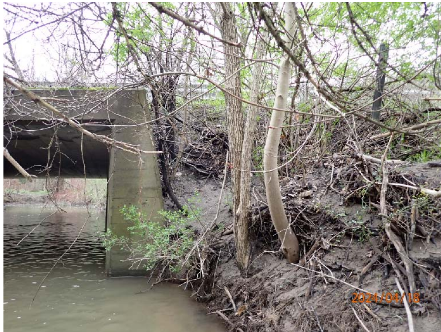
Photograph No. 4: 0690: Area of erosion at northeast corner.
