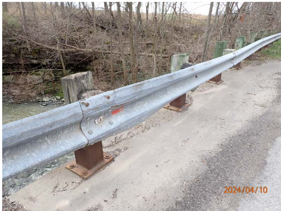
Photograph No. 4: 0142: Damaged guiderail over east side of the structure.
