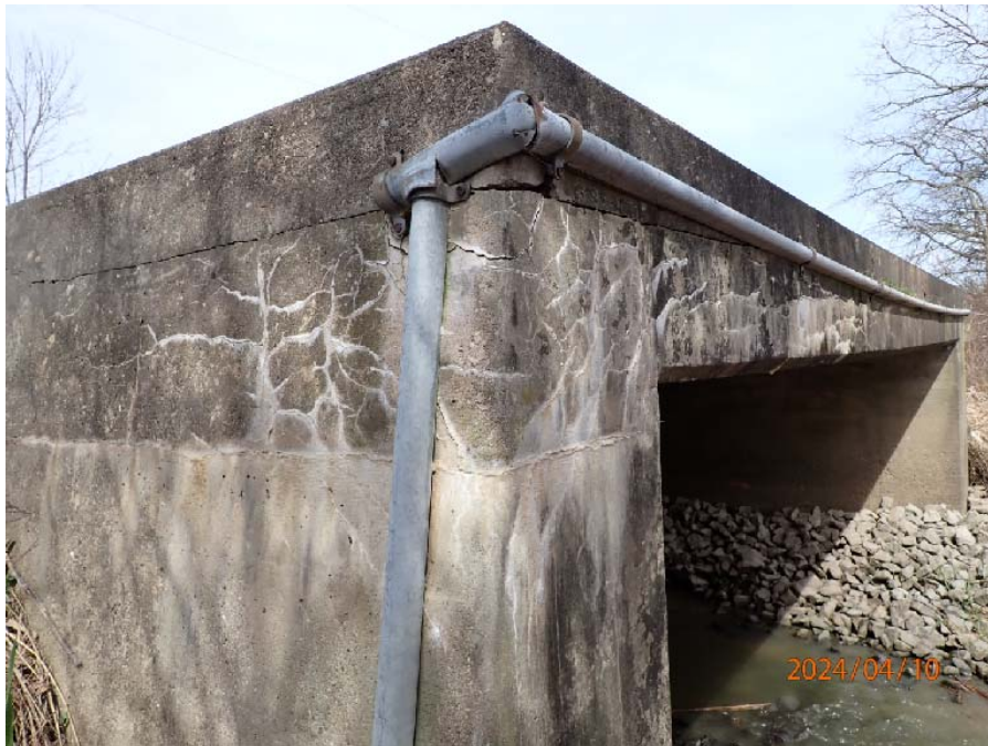
Photograph No. 4: 0374: Cracking and efflorescent staining at southeast corner.
