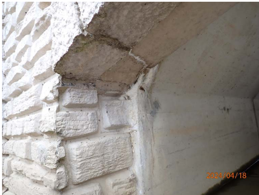
Photograph No. 4: 0113: Leakage and efflorescent staining at southwest corner.
