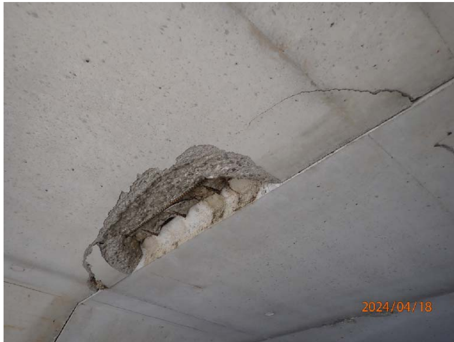
Photograph No. 4: 0034: Spall in precast unit at east end.
