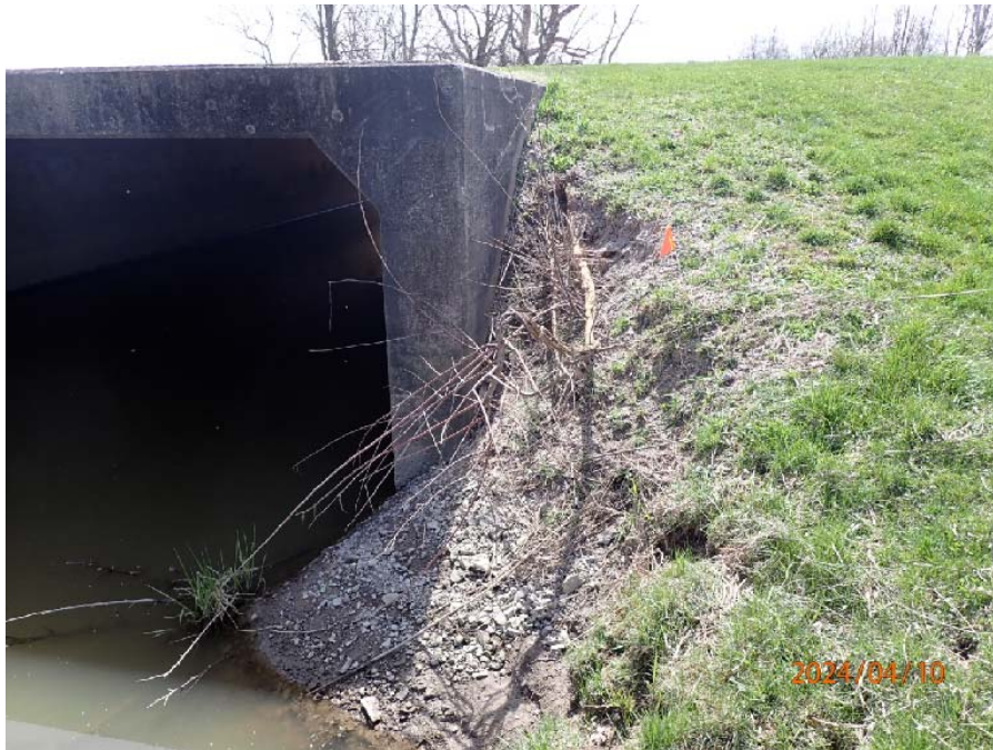
Photograph No. 4: 0523: Erosion at northwest corner.
