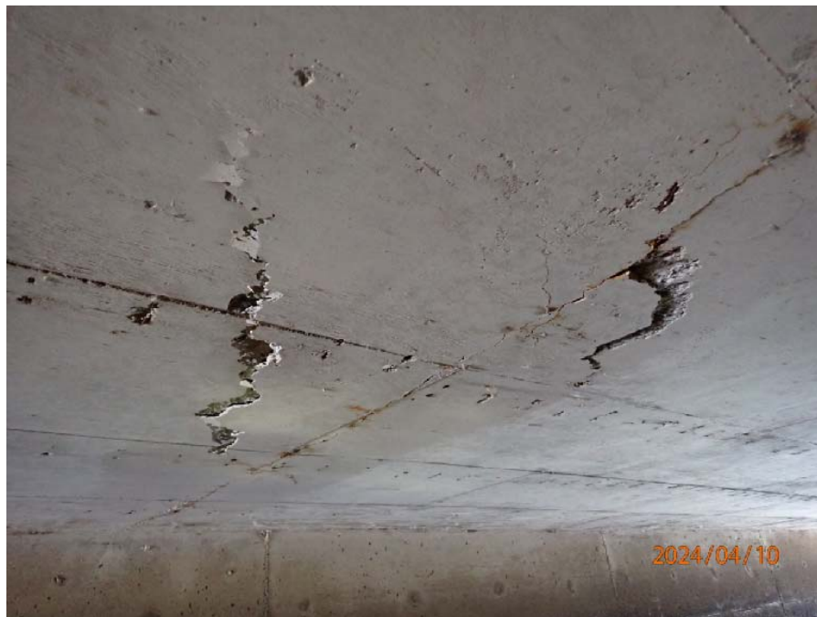
Photograph No. 4: 0259: Delamination at midspan.
