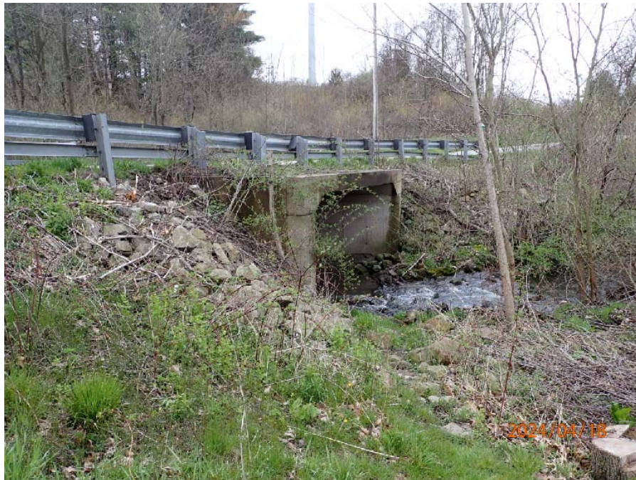
Photograph No. 2: 0214: South elevation and erosion at southwest corner.
