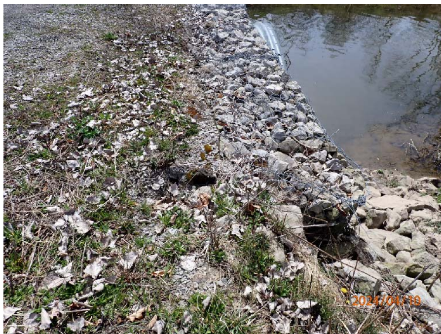
Photograph No. 4: 0611: Gabion basket at northwest corner with loss of stone.
