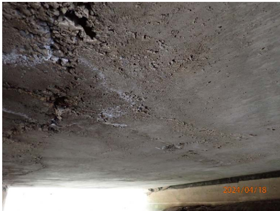
Photograph No. 4: 0493: Area of delamination in the soffit at centre span.
