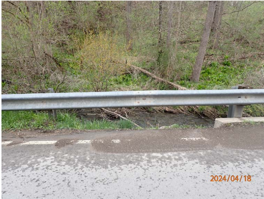
Photograph No. 4: 0286: Missing guiderail post at southwest corner.
