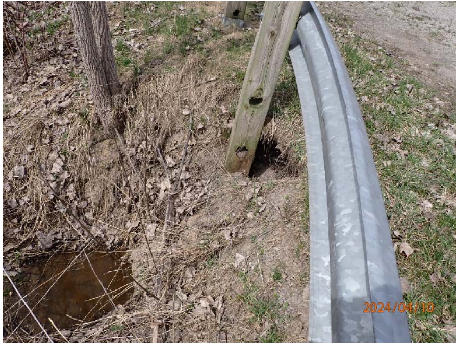
Photograph No. 4: 0402: Sinkhole at driveway rounding at northwest corner.
