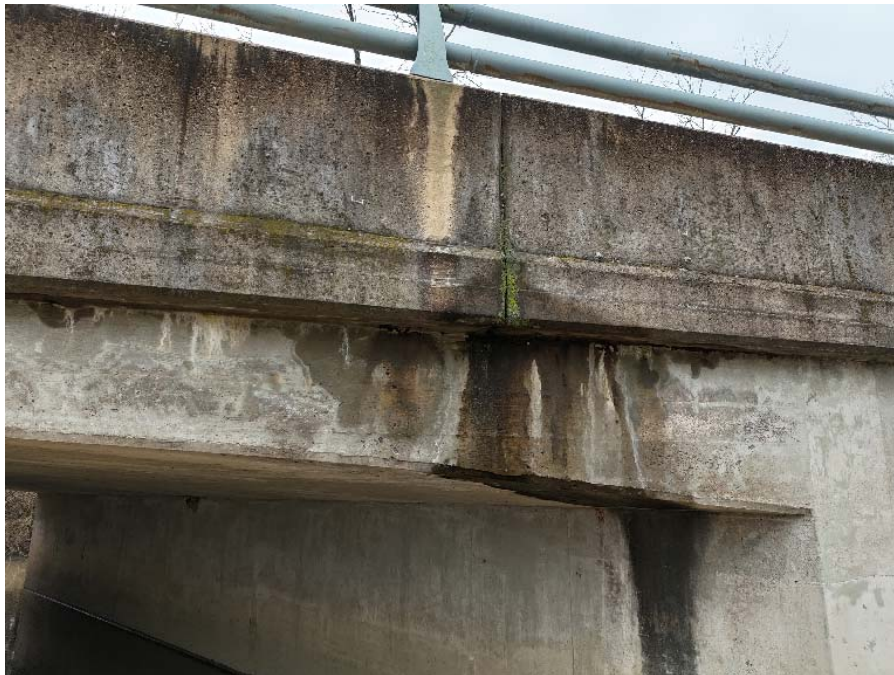
Photograph No. 4: DJI_0009: Leakage in west fascia looking northeast.
