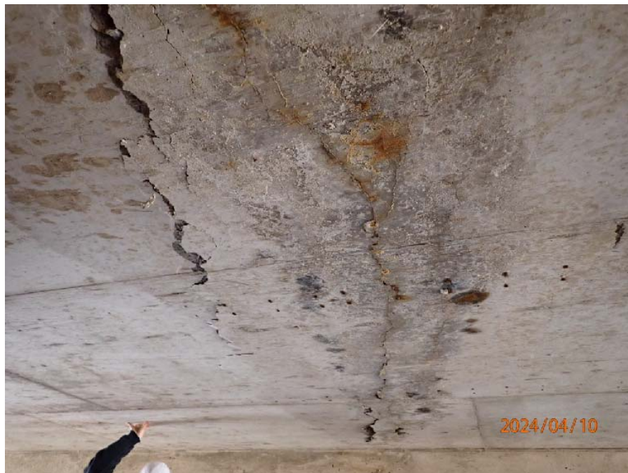
Photograph No. 4: 0307: Area of delamination and spalling 2m west of center.
