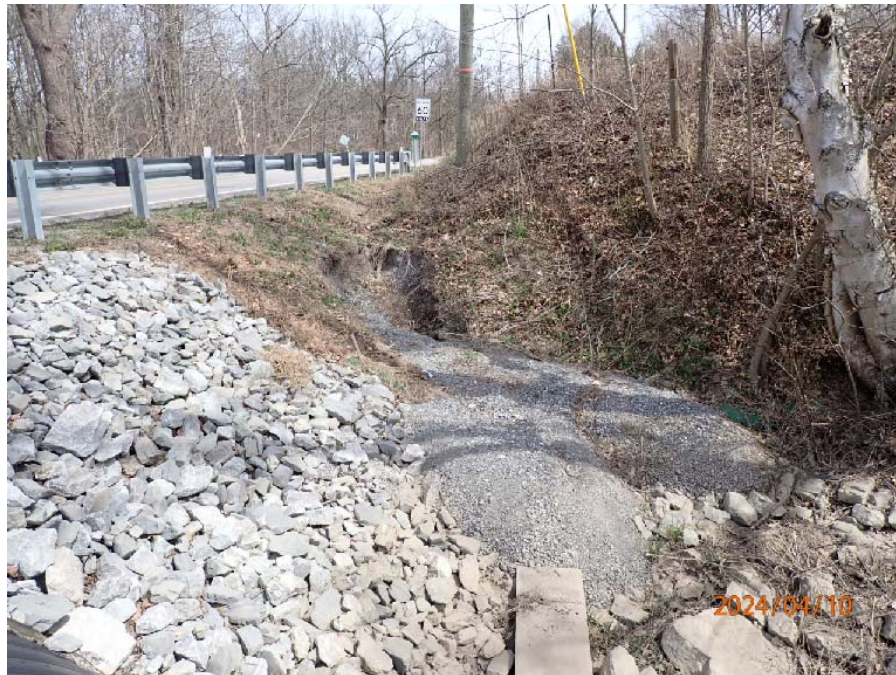
Photograph No. 4: 0677: Area of granular washout at southeast corner.
