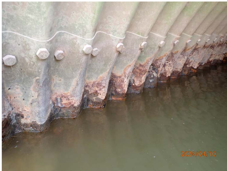
Photograph No. 4: 0797: Severe corrosion along the waterline (typical).
