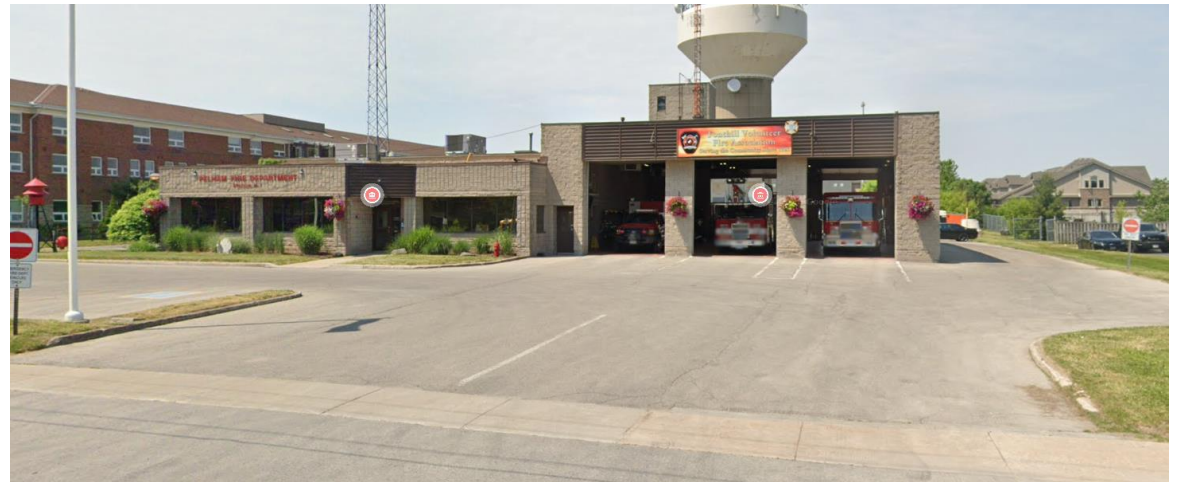
Figure 2 –Existing Building – Town of Pelham Fire Station 1
