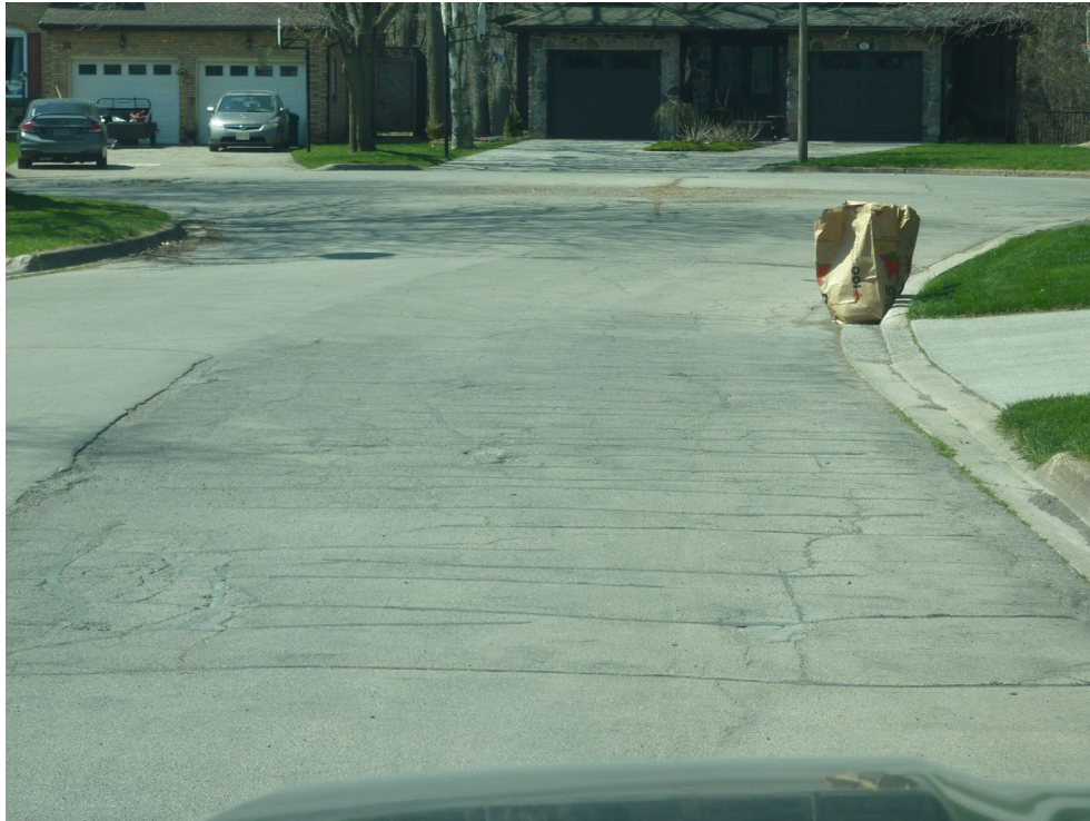
Figure 2-5. Section 456.01, Beechnut Court, from Berkwood Place to End – HCB (Poor Condition, PCI = 50)
