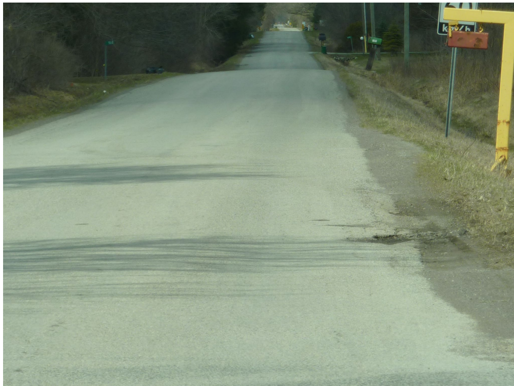
Figure 2-6. Section 211.04, Sumbler Road, from Cream Street to Centre Street – LCB (Good Condition, PCI = 70)
