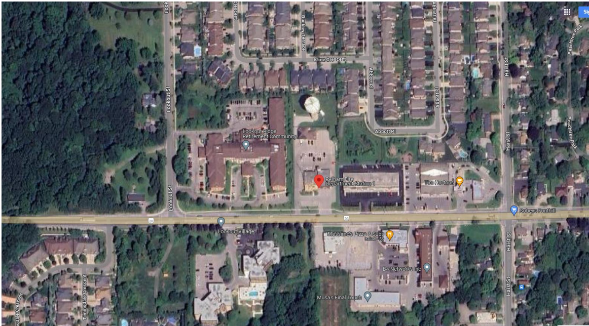
Figure 1 –Existing Site– Town of Pelham Fire Station 1
