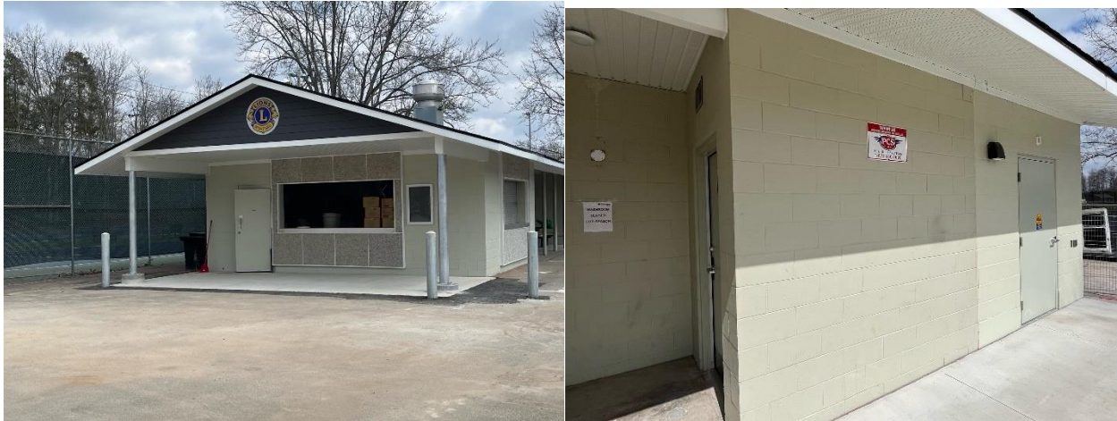
Completed Centennial Park Concession and Washrooms
