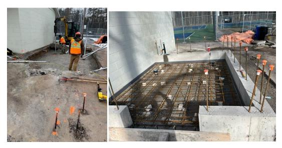
Helical Pile Installation and Completed foundation ready for concrete slab.
