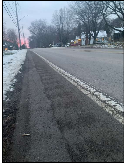
Figure 3.4 – Eroded Rumble Strips
