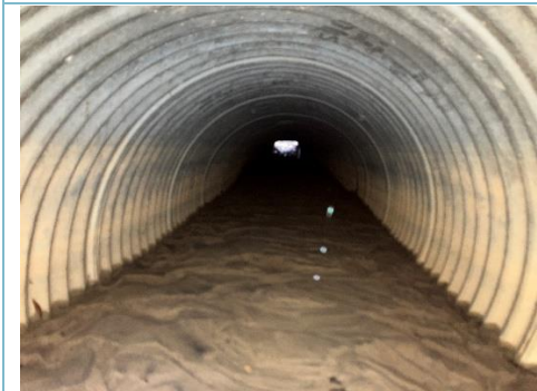
Upstream culvert 25% full with sand (deficiency)
