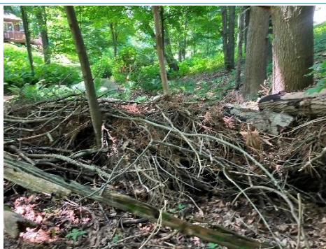
Blockage along outflow path (deficiency)
