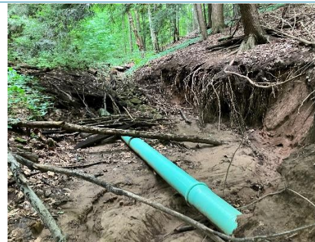
Exposed Sanitary Pipe in low flow channel (deficiency)
