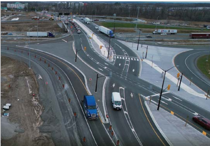
Diverging Diamond Interchange under construction in December 2022
