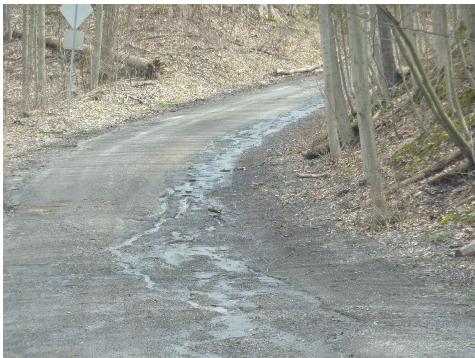
Figure 2-11. Section 121.01, Luffman Drive, from Sulphur Spring Drive to Orchard Hill Road – LCB (Poor Condition, PCI = 46)
