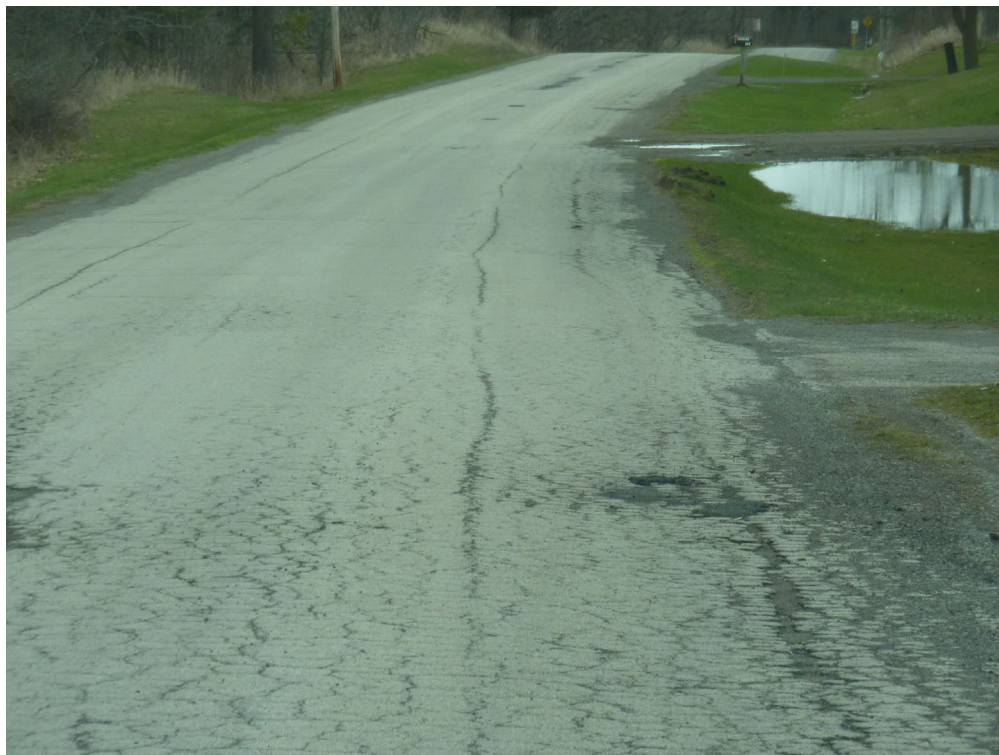
Figure 2-10. Section 114.06, Roland Road, from Effingham Street to Sulphur Springs Drive – LCB (Fair Condition, PCI = 54)
