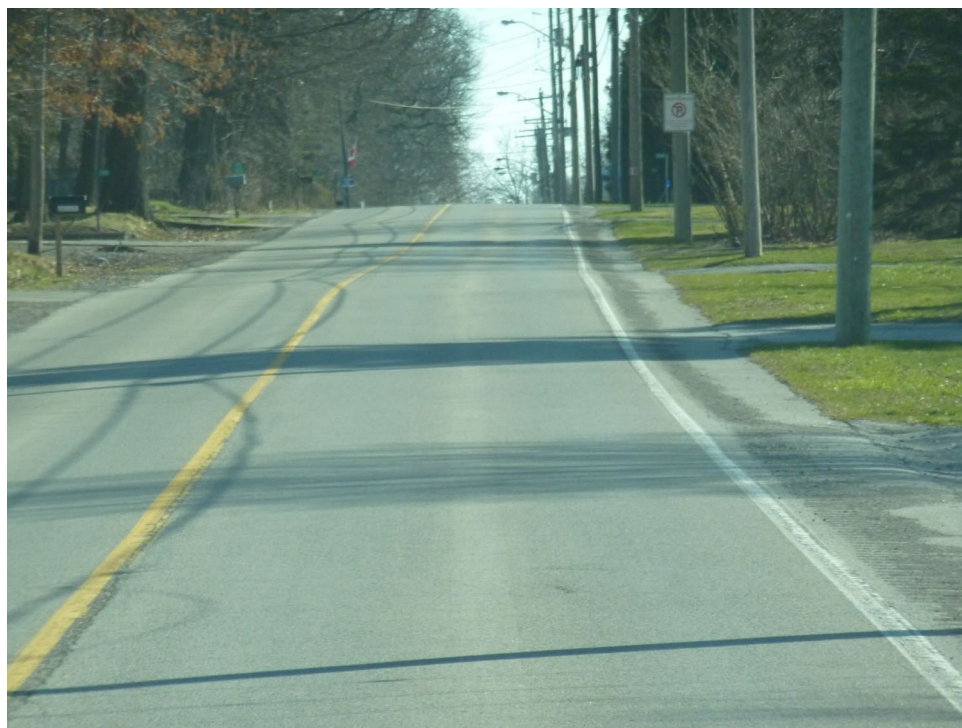
Figure 2-6. Section 420.07, Canboro Road, from Effingham Street to Oakridge Boulevard – HCB (Good Condition, PCI = 72)
