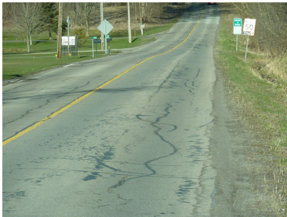
Figure 2-7. Section 206.06, Welland Road, from Centre Street to Effingham Street – HCB (Fair Condition, PCI = 56)
