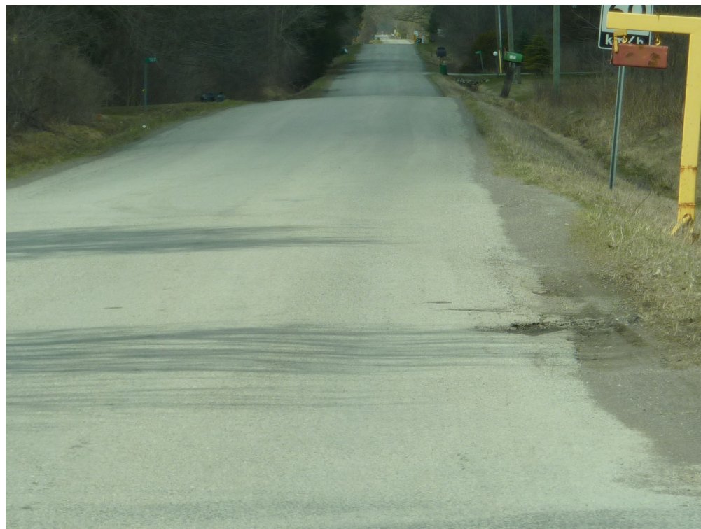
Figure 2-9. Section 211.04, Sumbler Road, from Cream Street to Centre Street – LCB (Good Condition, PCI = 70)
