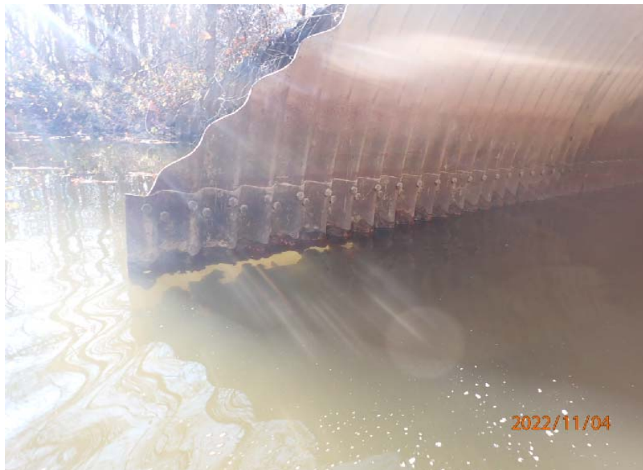
Photograph No. 4: 0294: Severe corrosion and perforations along north side of south cell.
