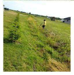
FLOW OBSTRUCTION due to High Vegetation along the Crossings and Open Channels
