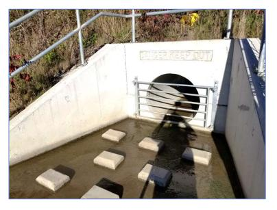
Figure : Existing undersized Culvert under Victoria Road
