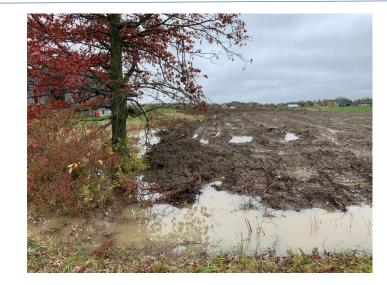
View from the road, drainage issues and fill placement at the 250 Farr St area development pushing water into the Farr Street Ditch
