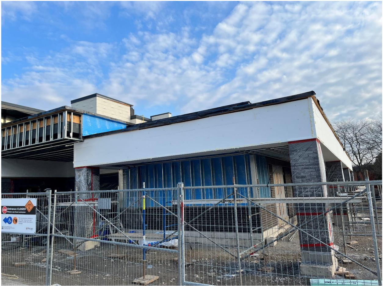
Building exterior with masonry and stucco, awaiting siding
