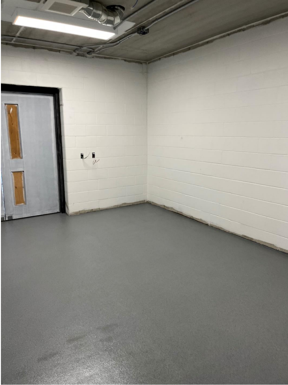
Epoxy floor installed
