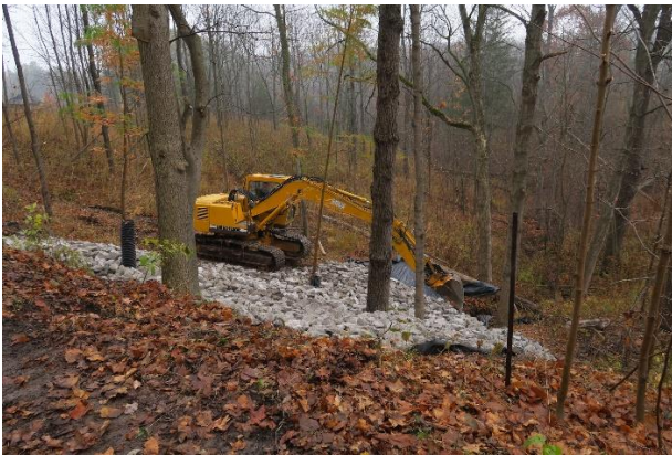
Photographs showing erosion treatment on the bank and road reconstruction using geo-reinforcement.
