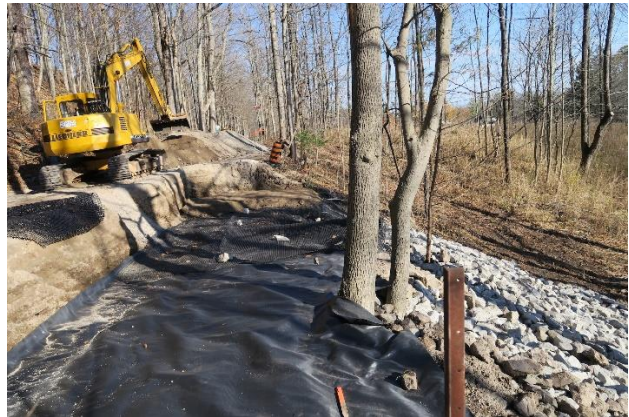
Photographs showing erosion treatment on the bank and road reconstruction using geo-reinforcement.
