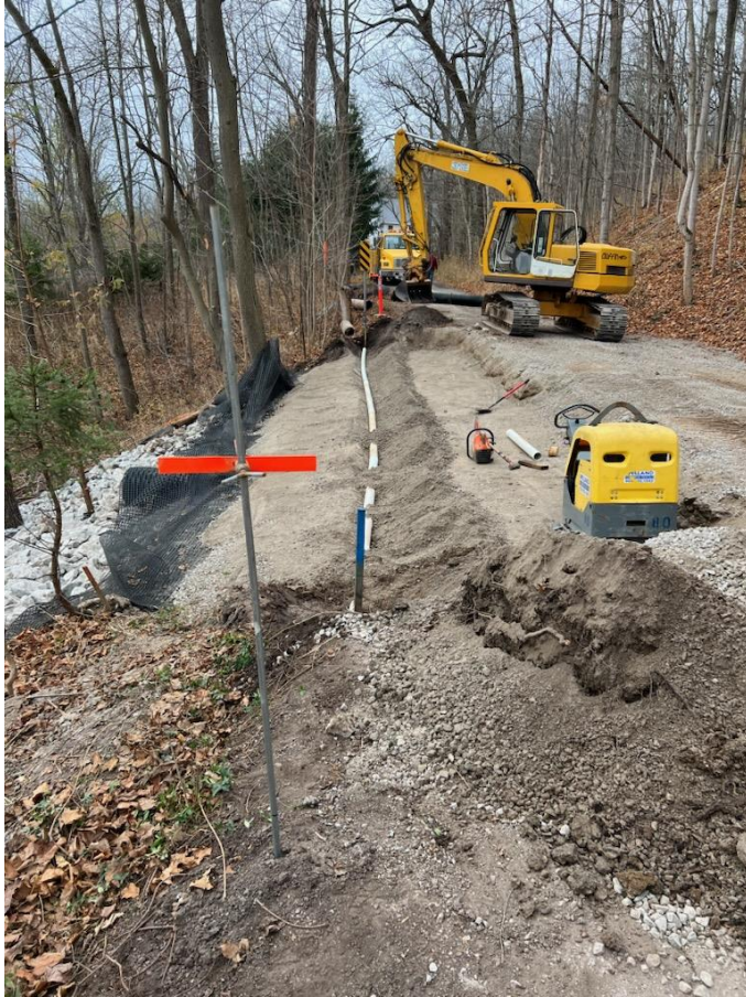
Photograph showing roadway reconstruction and backfill.
