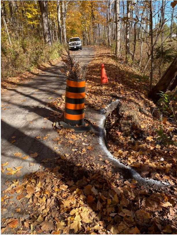
Photographs showing erosion and failure of the existing roadway.
