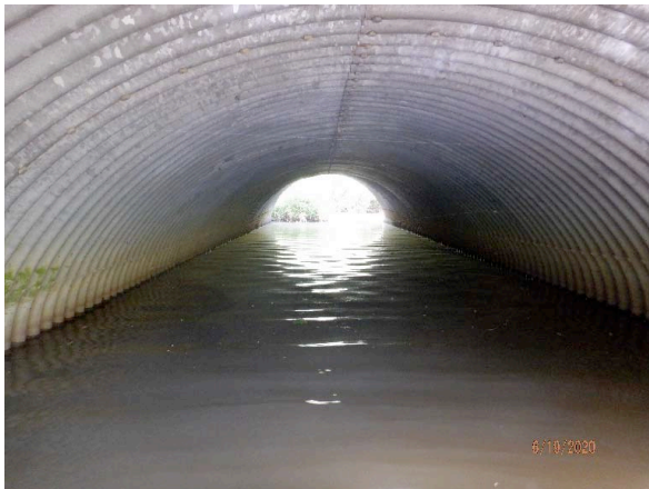
Figure 24. Interior of south cell, looking west.
