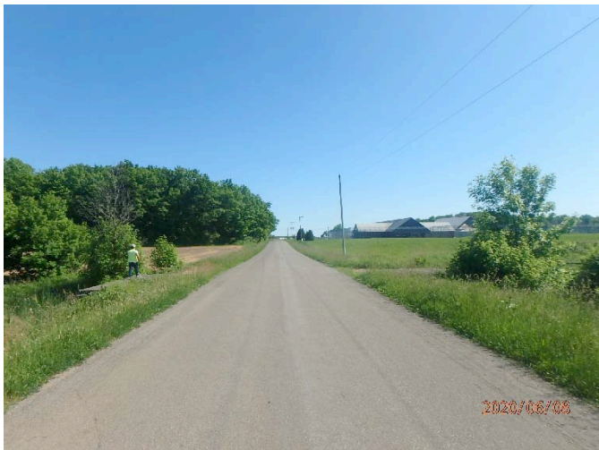
Figure 14. Surface treated roadway looking south.
