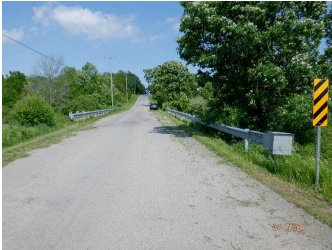
Figure 18. Roadway looking east.
