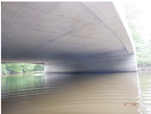
Figure 28. Interior looking northeast.
