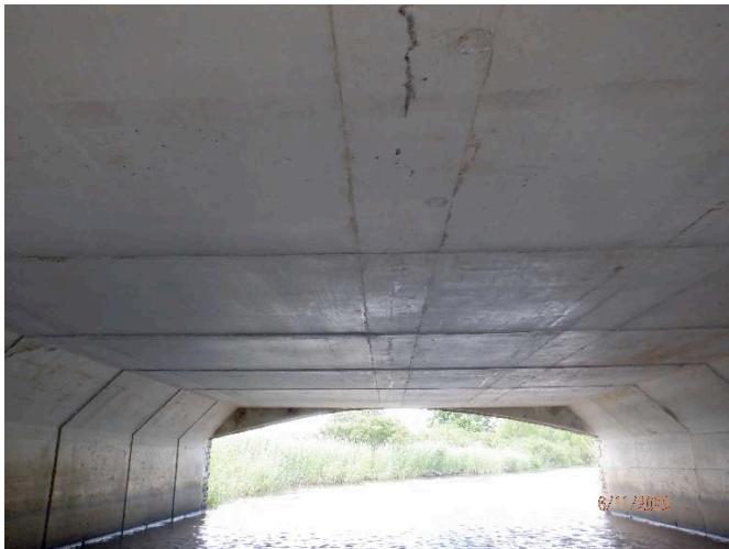
Figure 19. Interior of structure, looking north.
