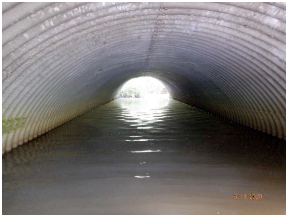
Figure 24. Interior of south cell, looking west.
