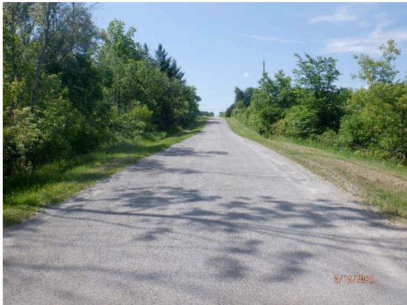
Figure 22. Roadway over structure looking south.
