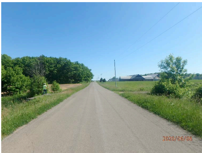
Figure 14. Surface treated roadway looking south.
