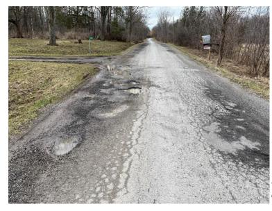
Road Base Failure and pavement deterioration on Roland Road
