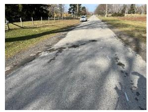
Tice Road: Road Base Failure
