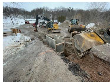
Installation of new 6 inch watermain at MSSP.
