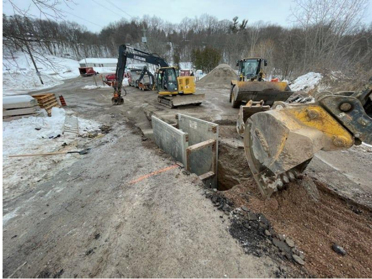
Installation of new 6 inch watermain at MSSP.
