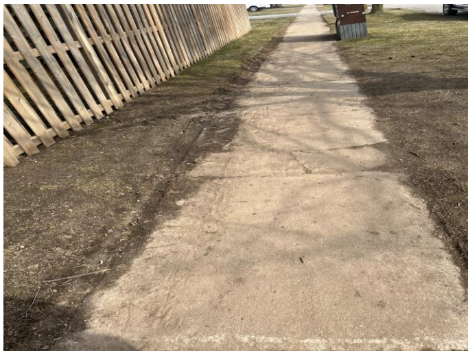
Sinking panels at Lawrence Lane
