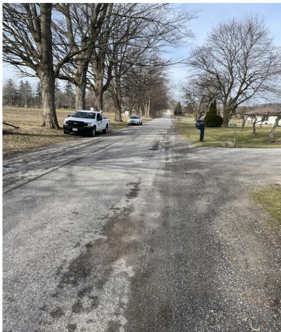
Tice Road Failing Road Shoulders
