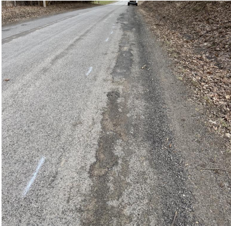
Metler Road: Road Shoulder Failing
