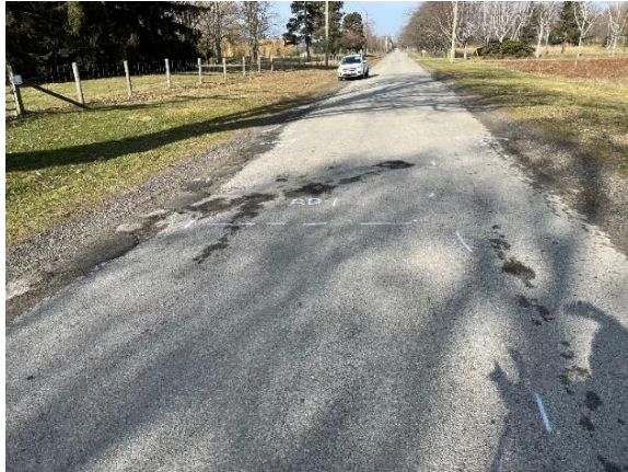
Tice Road: Road Base Failure
