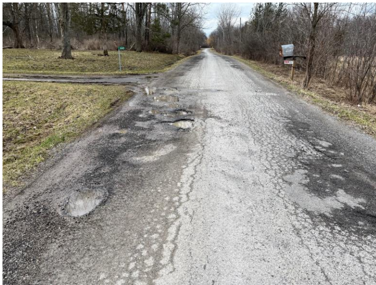
Road Base Failure and pavement deterioration on Roland Road
