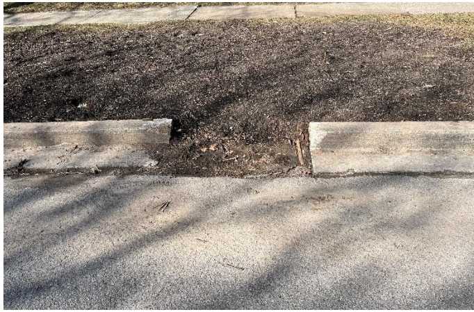
Missing curb at Millbridge
