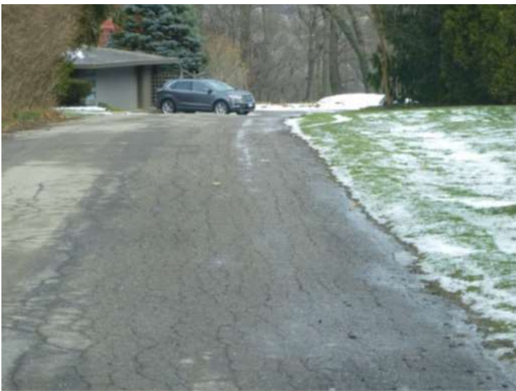
Figure 7. Spencer Lane, from Pinecrest Court to End – HCB (Poor condition, PCI = 49)
