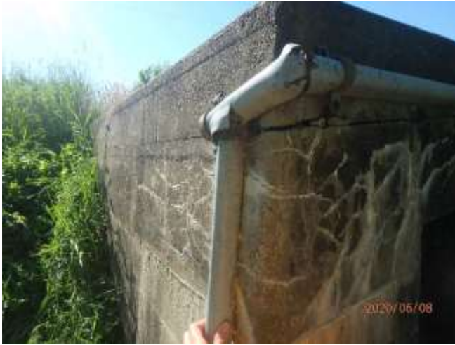
Figure 16. Wide horizontal crack at south east corner.
