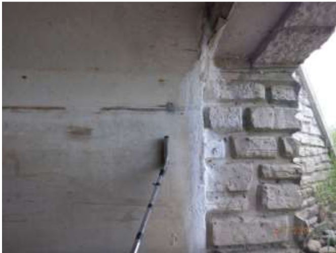
Figure 20. Leakage and efflorescent staining at northwest corner.
