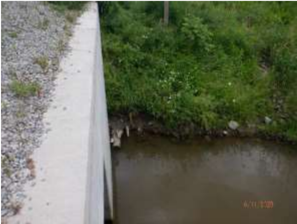
Figure 29. Erosion at southeast corner.
