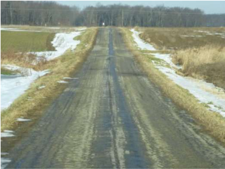
Figure 11. Balfour Street, from River Road to Webber Road (RR29) – LCB (Poor condition, PCI = 47)
