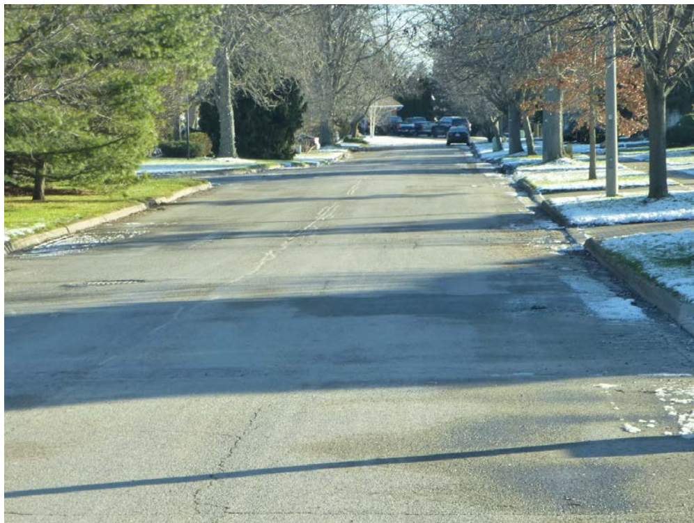
Figure 2-6. Section 501.01, Kevin Drive, from Haist Street to Sherrilee Crescent – HCB (Fair Condition, PCI = 55)
