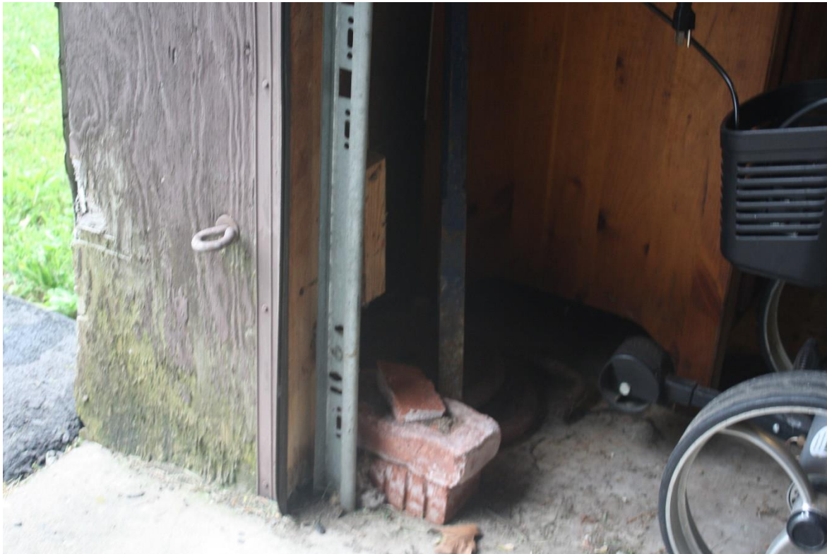
Figure 6: Interior Support Beam Rot
