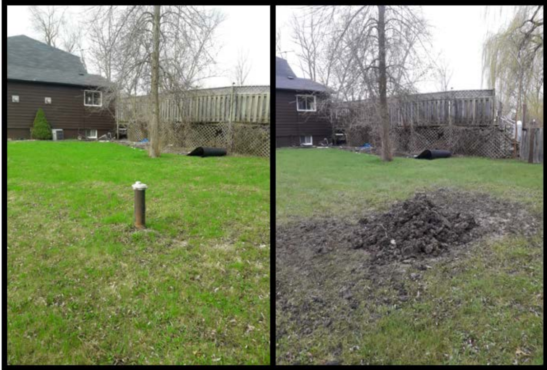
Figure 12: An example of a NPCA Water Well Decommissioning Project. Left photo shows an abandoned drilled well in need of decommissioning and the right photo shows same dug well after decommissioning had been completed by a licensed well contractor.
