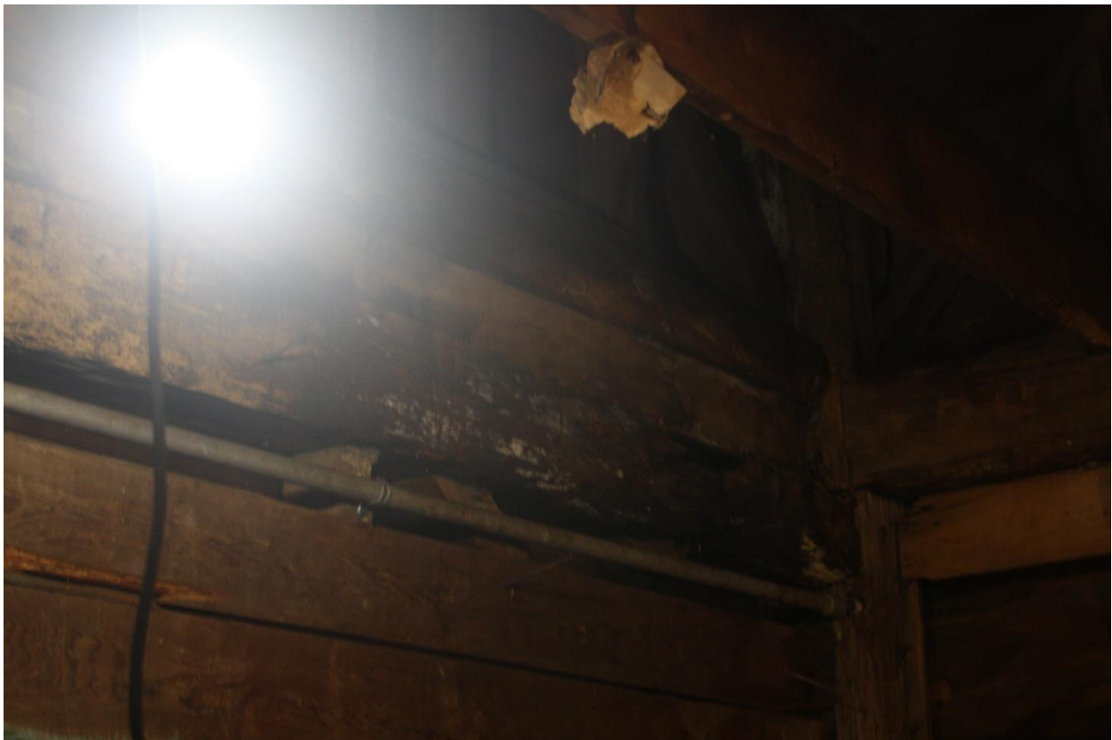
Figure 6: Interior Support Beam Rot
